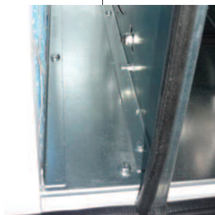
Figure I2b: Removable fanplate for supply fan removal.
