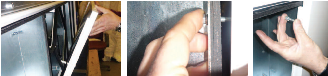
Figure 11a, 11b and 11c: Remove non control centre side access panel by removing the four bolts (2 x 2) on rear of panel and disconnect condensate pipe.
